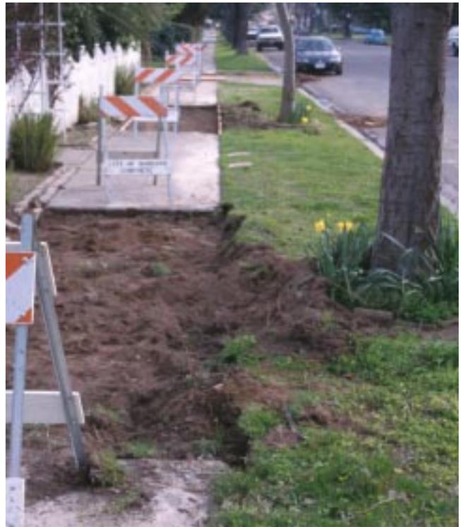
**Figure 1.** Sidewalk damage caused by tree roots is commonly found in California. Annual repair costs are substantial.
