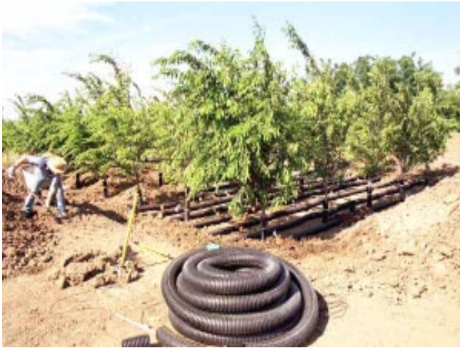
Figure 2. In the fill + aeration treatment, perforated pipe was placed on top of the field soil and between plot trees. Fill soil (12 inches) was then added on top of the aeration pipe and compacted to 1.6 g cc -1 .
