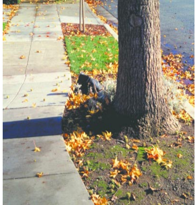
Avoiding shallow tree root damage by redirecting the sidewalk path. (Fig. 3)
